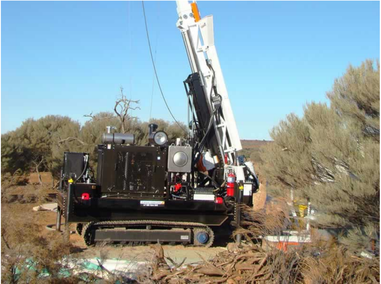
Typical Track Mounted Core Drill
